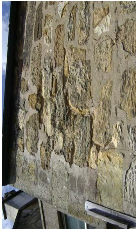
*Cement over pointing causing rapid masonry erosion*
