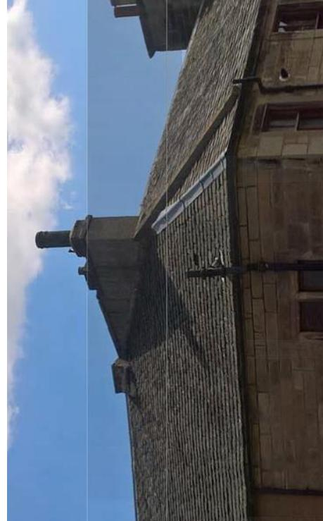
*Truncated and cement harled masonry chimney stack*
