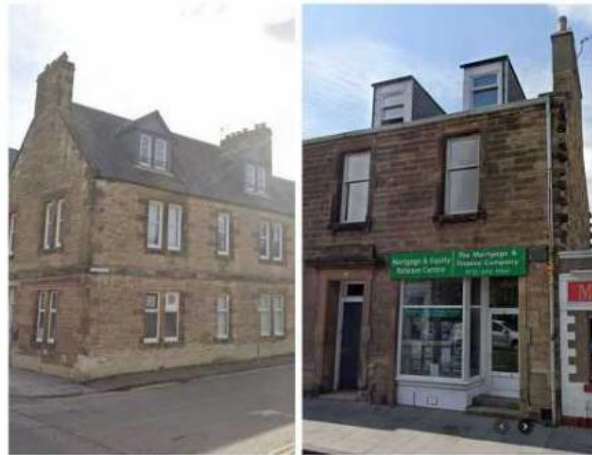
Photos of Dormer and Roof Extension Opposite and within Site Line of the Application Site
