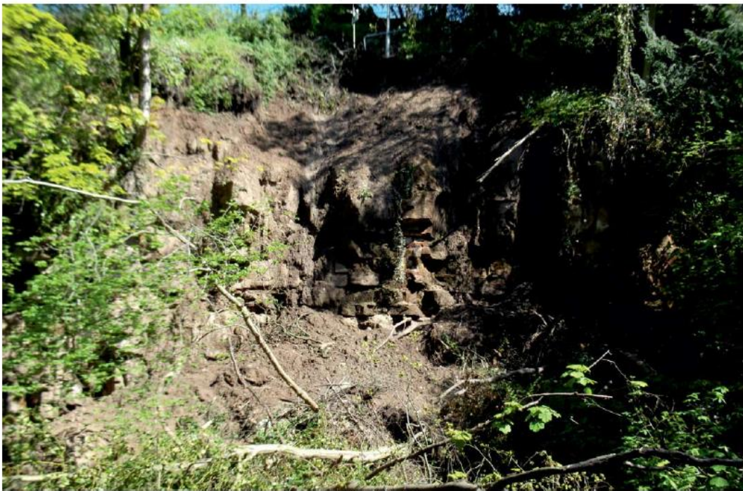
Photo 20. Washout at rock face / lower slope (23.04.16).
