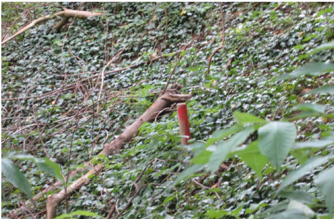
Photo 4. Marker post out of plumb.
