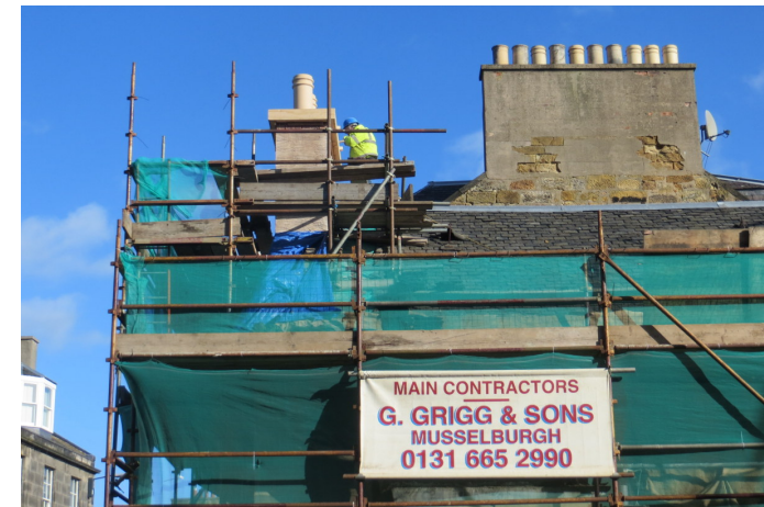
Serious deterioration of stonework in chimneystacks proved to be a characteristic problem encountered in many of the THI/CARS building improvements
