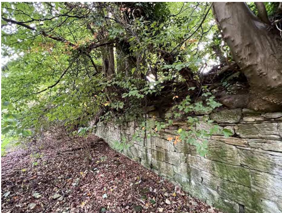
Photographic plate showing the old retaining wall. The road is above. The rooting areas of these trees are extremely complex.
