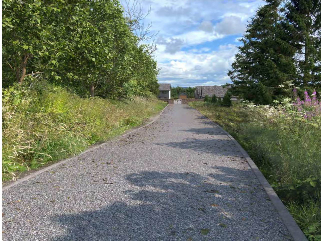
Fig 6: Illustrative Visualisation 2 of the proposed development viewed from the site access to the west. Visualisations shows the application site in real world profile, roofs of proposed dwellings can be seen to be most prominent feature.
