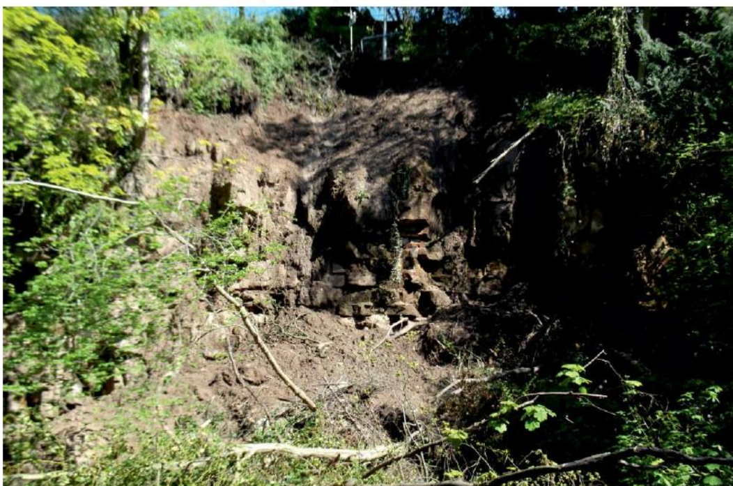
Photo 20. Washout at rock face / lower slope (23.04.16).
