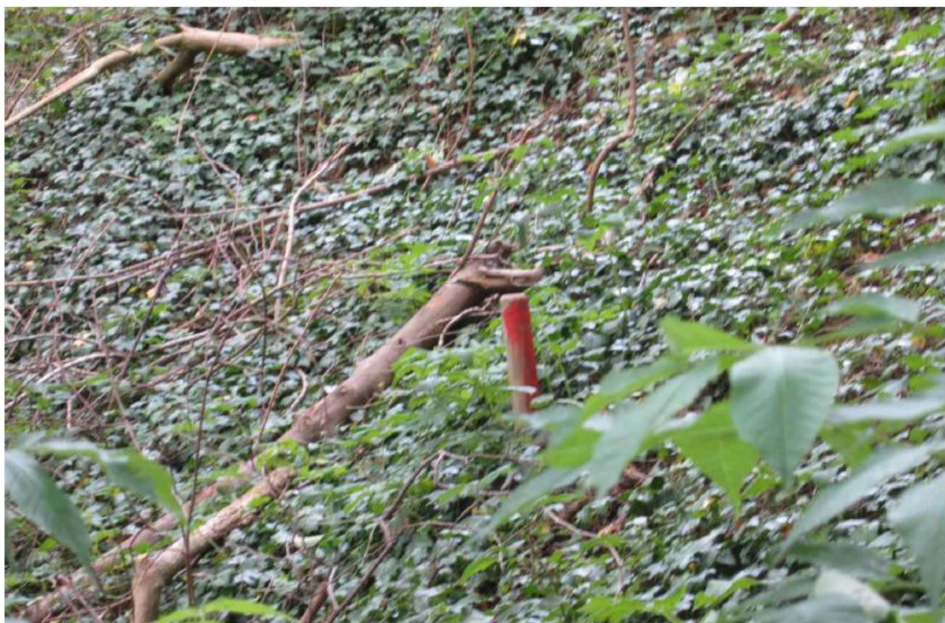
Photo 4. Marker post out of plumb.
