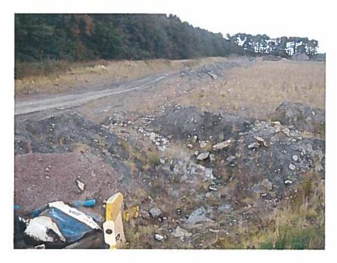
Photo 3: Pit into which drainage flows. There is no outlet from pit. There are at least 3 other pits of a similar type on the Pile Test Site.
