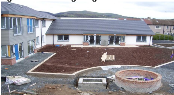
Figure 9.1: Building Progress at Extra Care Housing in Penicuik Project
