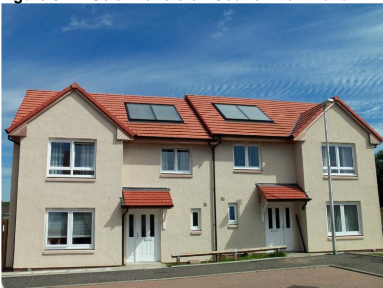
Figure 8.1 – Solar Panels on Council New Build
