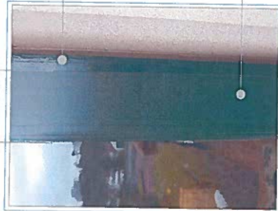
Upvc Sample - photographed inline with existing frames Please note; Proposed UPVC profile matches frame width of existing Timber Windows
