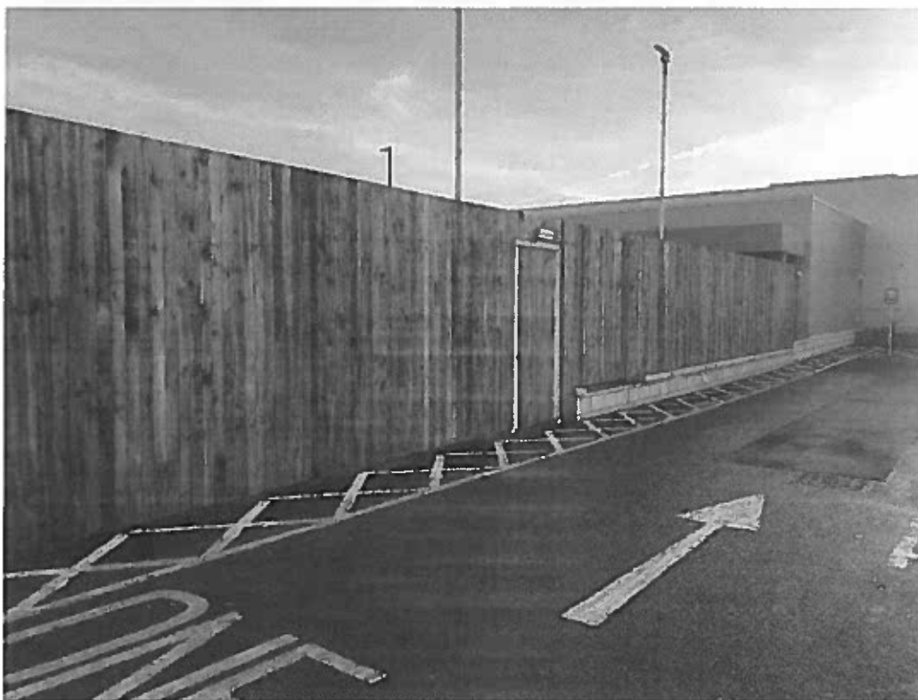
Figure 1: Fence from north-west of the site.
