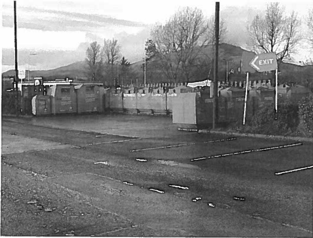
Figure 8: Use of timber palisade fencing within the recycling area of the Sainsbury's store.
