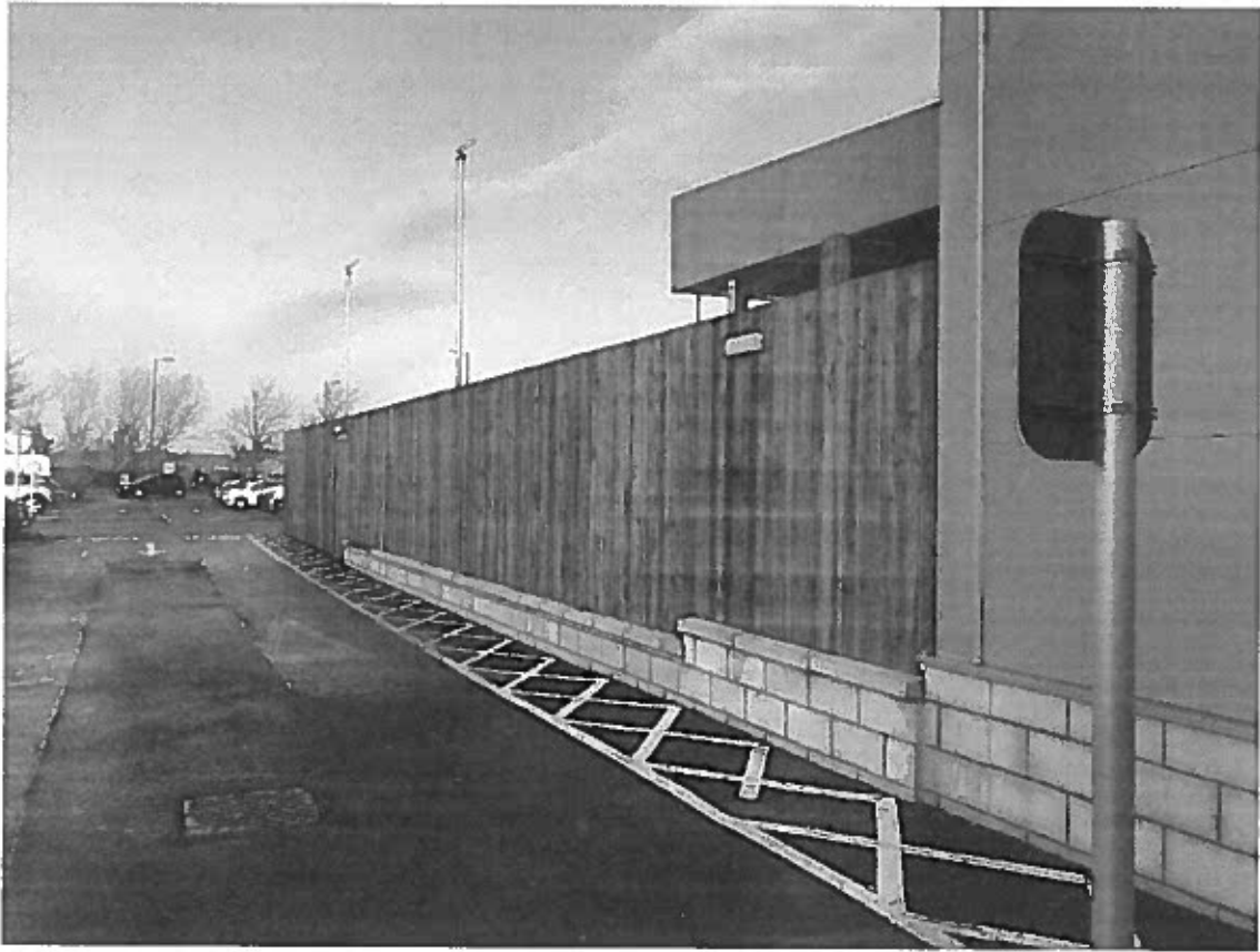
Figure 3: Fence from south west of site.
