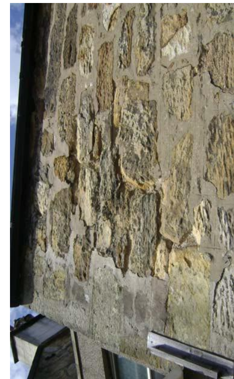
Cement over pointing causing rapid masonry erosion
