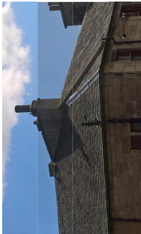
Truncated and cement harled masonry chimney stack
