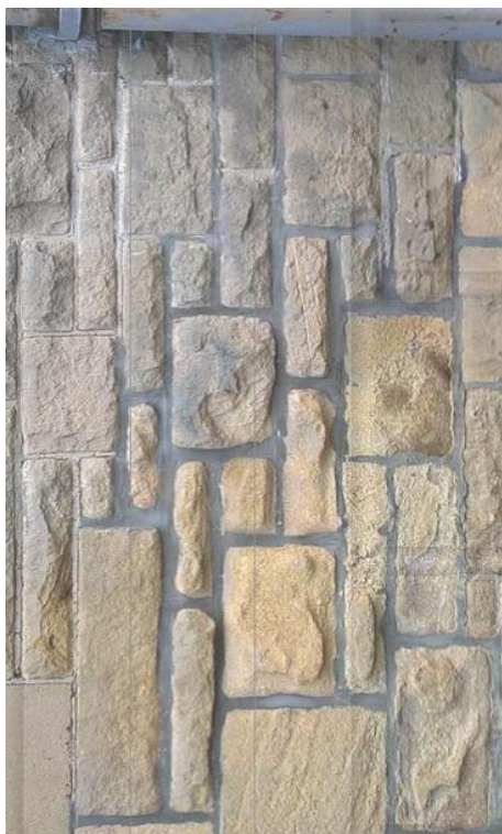
Evidence of recent cement pointing
