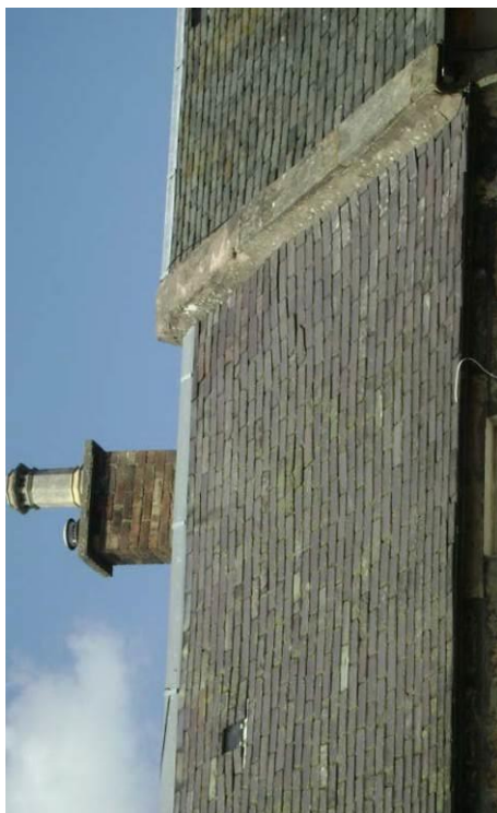
Welsh slate roof showing numerous patch repairs West Street
