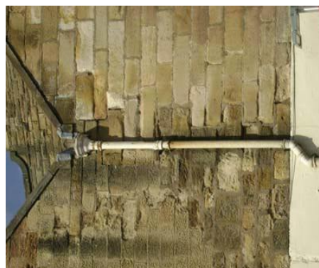
Water damage to masonry
