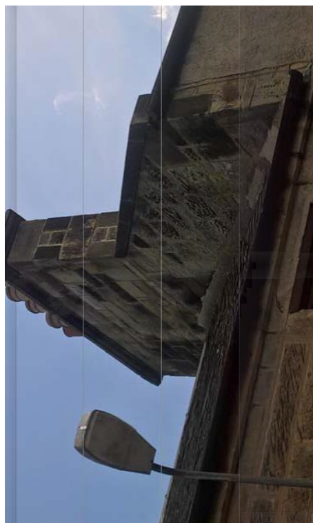
Failed cement fillet at base of gable and junction with slates
