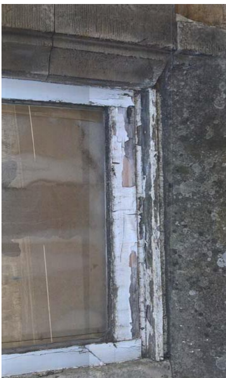
Evidence of lack of maintenance of paintwork on West Street
