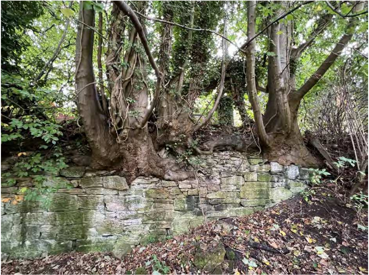
Photographic plate showing the old retaining wall. The road is above and the occluded stems of trees T82 and T83 can be seen growing out of the wall. The rooting areas of these trees are extremely complex.
