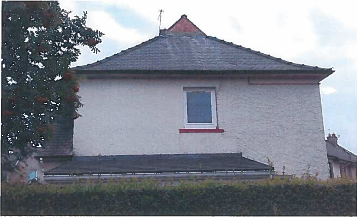
Existing Roof finishes 2019
