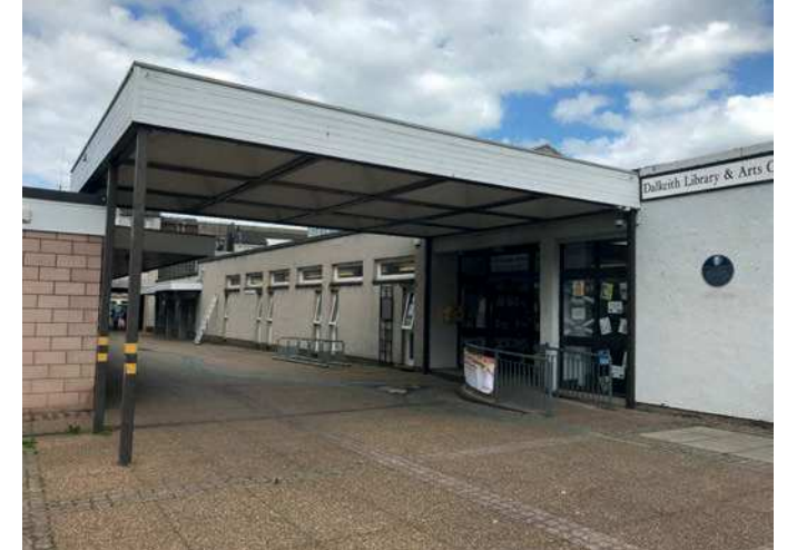
Dalkeith Library - The library facilities and arts centre have no active frontage.
