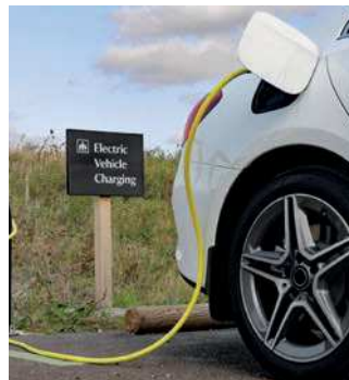
Fig.26 Electric vehicle charging points nationaltrust.org
