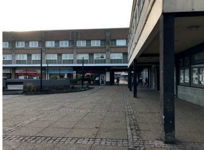
Eskdail Court - Buildings and townscapes in a poor state of repair and lack of green space in the public realm.
