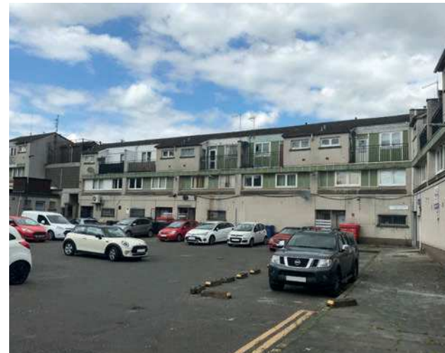
Eskdail Court - Housing overlooking car park and service access. Housing lacks amenity space and are in poor condition.
