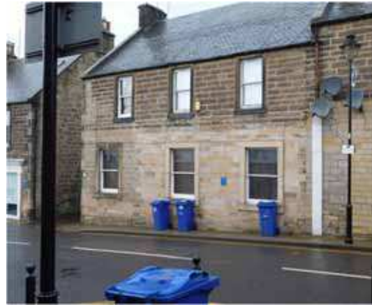
Illustration 2: New stone infill still not blending in with the old.
