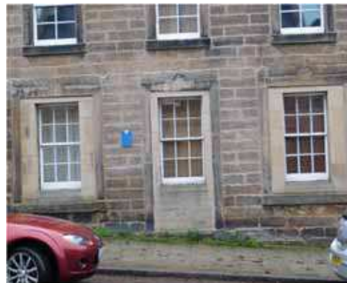
Illustration 4: Stone infill to doorway
