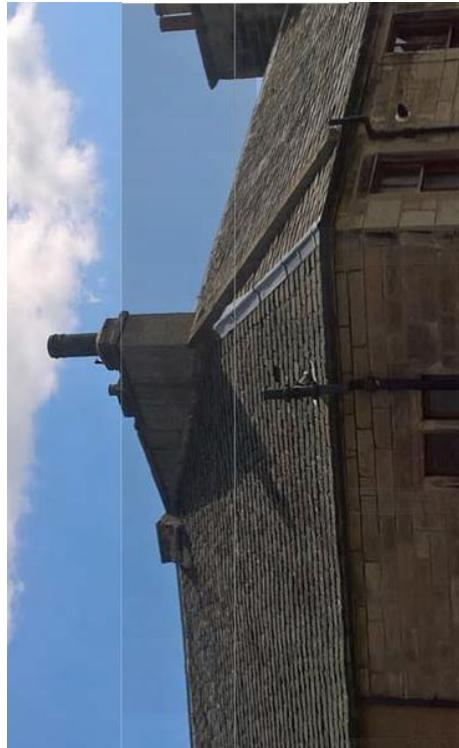
*Truncated and cement harled masonry chimney stack*
