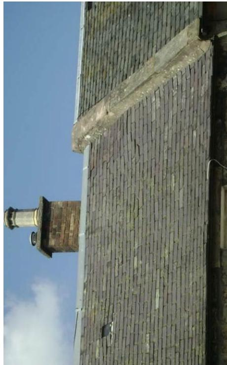
*Welsh slate roof showing numerous patch repairs West Street*
