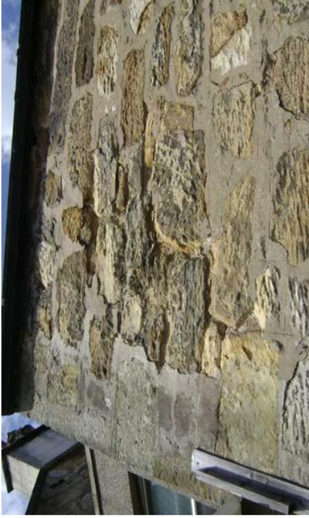
*Cement over pointing causing rapid masonry erosion*
